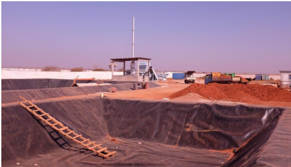
Figure 65: Ash mono-fill example
