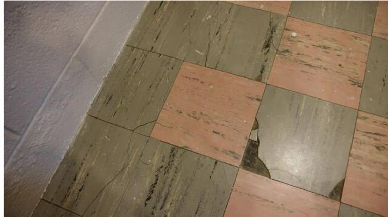
**Figure 67: Asbestos containing products**
