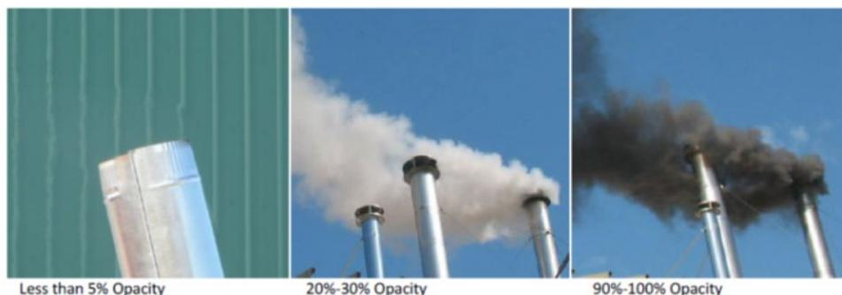
**Figure 8: Emission opacity indicating ideal or problematic incineration efficiency**
