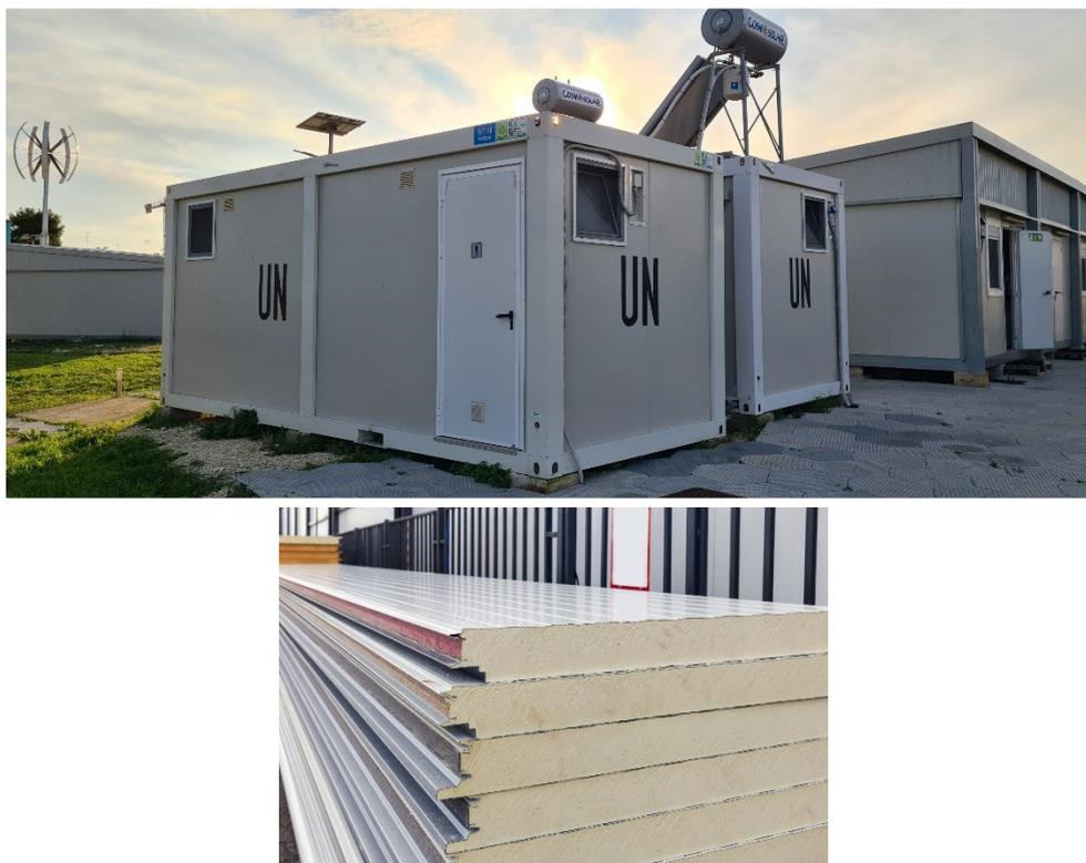
**Figure 19: Prefabricated building and panel with PUR/PIR insulation**
